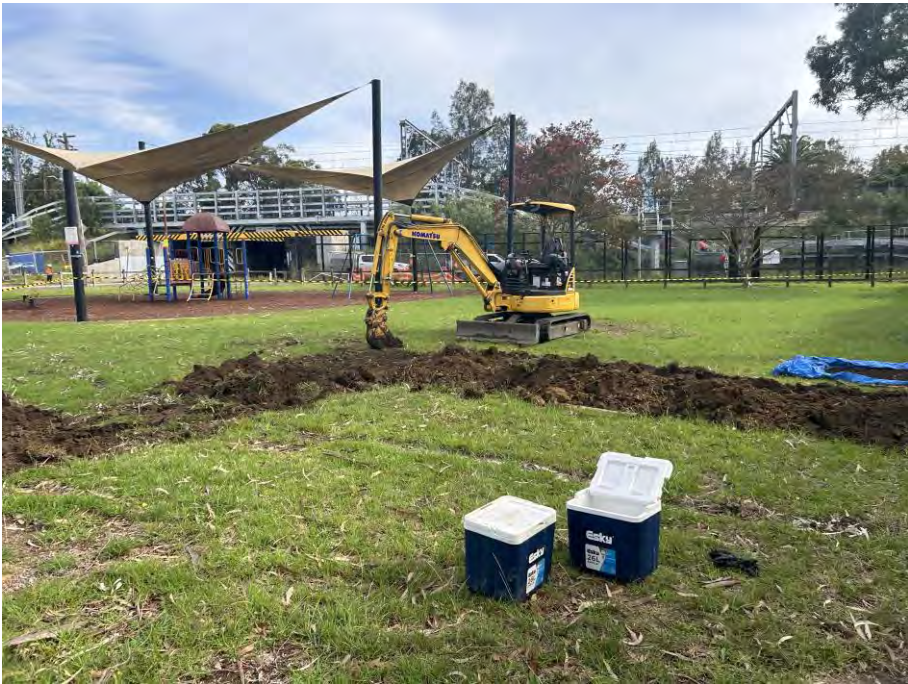
Image 9.1.1.1 Photograph of excavator and strip trench.
